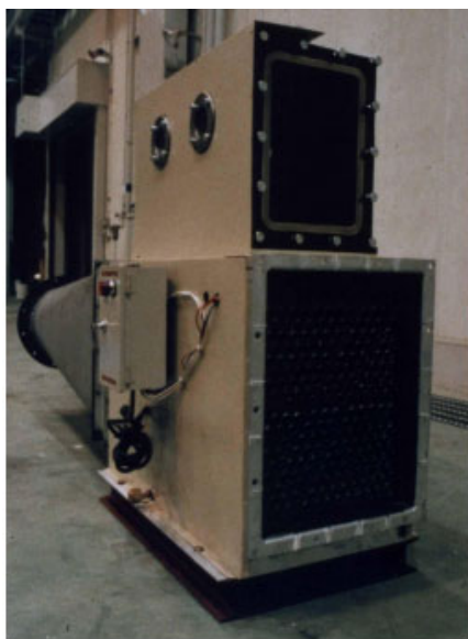
Fig. 6. Thermoelectric recuperator installed at the thermal power plant of the Tokyo Electric Power Company [106].
