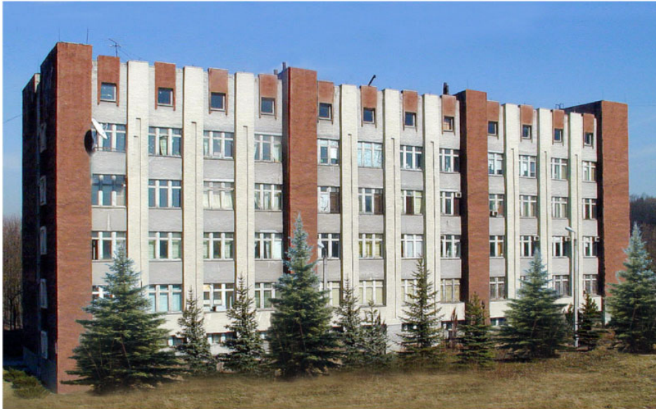
Laboratory building of Institute of Thermoelectricity
