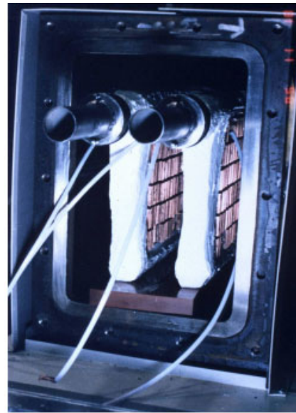
Fig. 6. Thermoelectric recuperator installed at the thermal power plant of the Tokyo Electric Power Company [106].
